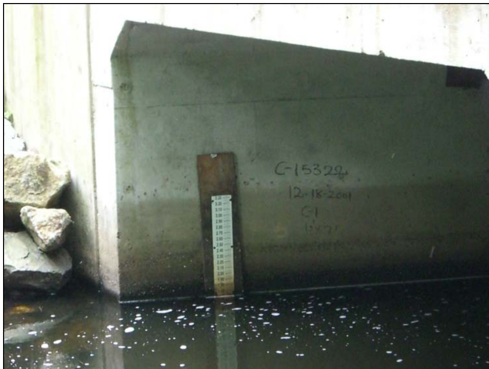
Photo 22 - The staff gauge located at the Catacunemang Road Bridge downstream of the dam.
