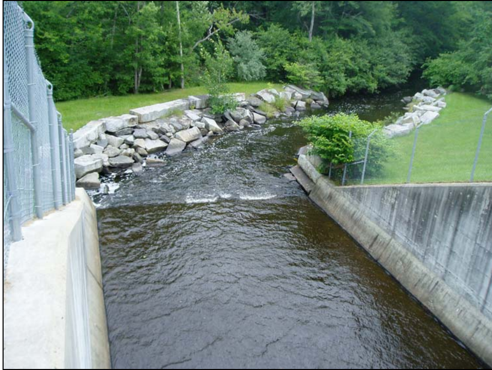
Photo 19 - The spillway discharge channel from the catwalk.
