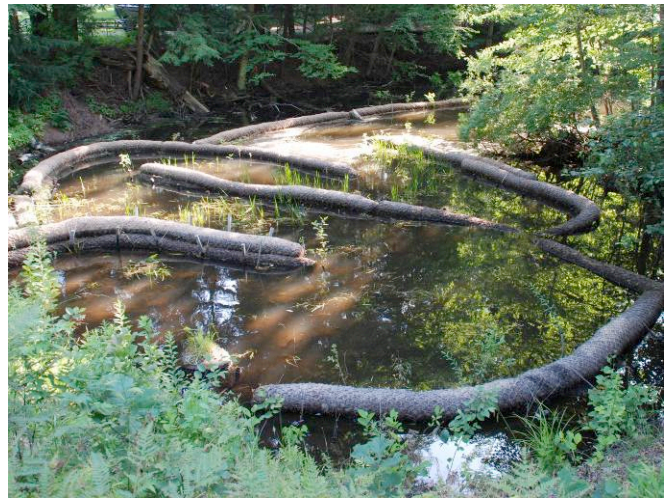
A degraded wetland area adjacent to a Lake Shirley tributary was restored with biodegradable coir fiber logs and plantings. Over time, the sinuous flow path will become densely vegetated to provide improved pollutant filtering and attenuation.
