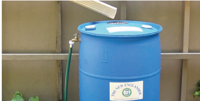
Rain barrel capturing roof runoff at the Acton Discovery Museum.
