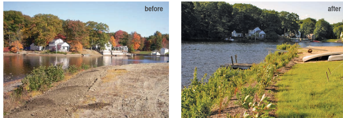
In 2008, a 400-foot shrub buffer was installed along the shoreline of Lake Shirley at the Oakes Landing subdivision. The buffer included 274 native shrub plantings, soil amendments and mulch.
