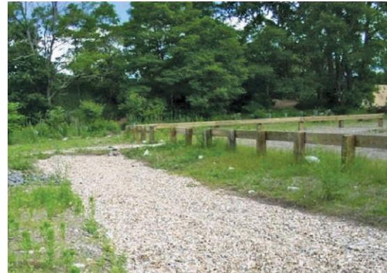
A stone infiltration trench designed to infiltrate stormwater from an adjacent parking area.
