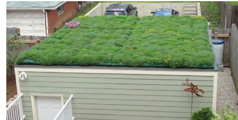
Roof gardens can be built almost any flat roof top, from residential to commercial to industrial. Photo credit: http://www.livegreencincinnati.com
